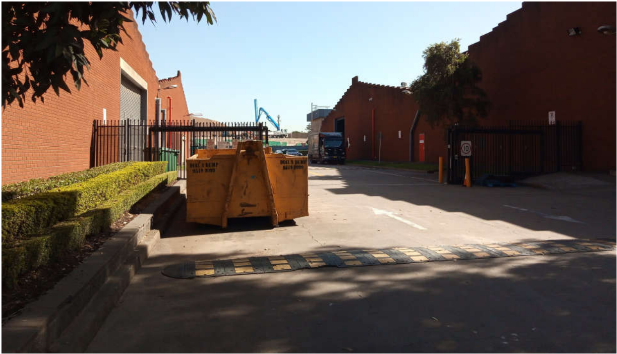
Photo 1 - General Site Conditions - Site Entrance
